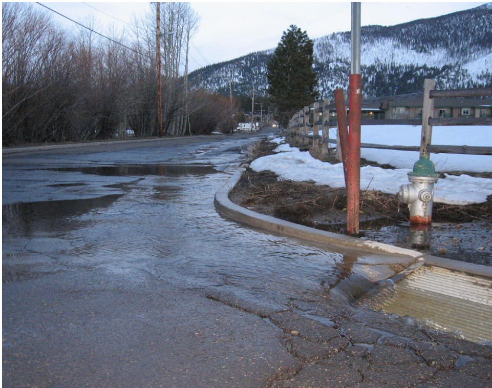
Existing stormwater issues on Kahle Drive
